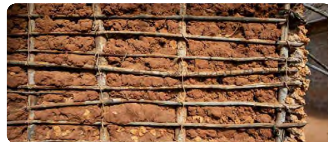
Traditional uses of mangroves such as the use of mangrove poles for home-building here in Mtangawanda, Kenya, can only be learned in a local context. © Sarah Waiswa
