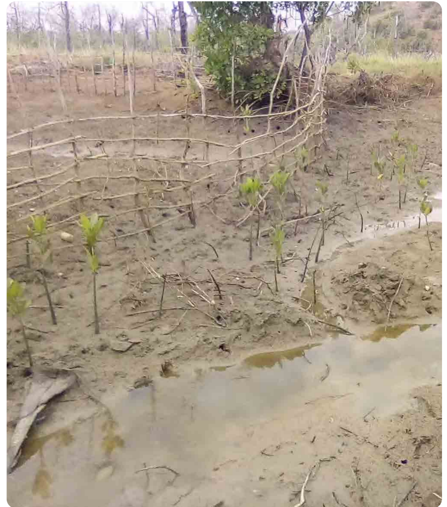
Community providing a solution to goat grazing stressor on mangroves by constructing a fence using local materials without obstructing the water hydrology to the mangrove. © Gilbert Atuga
