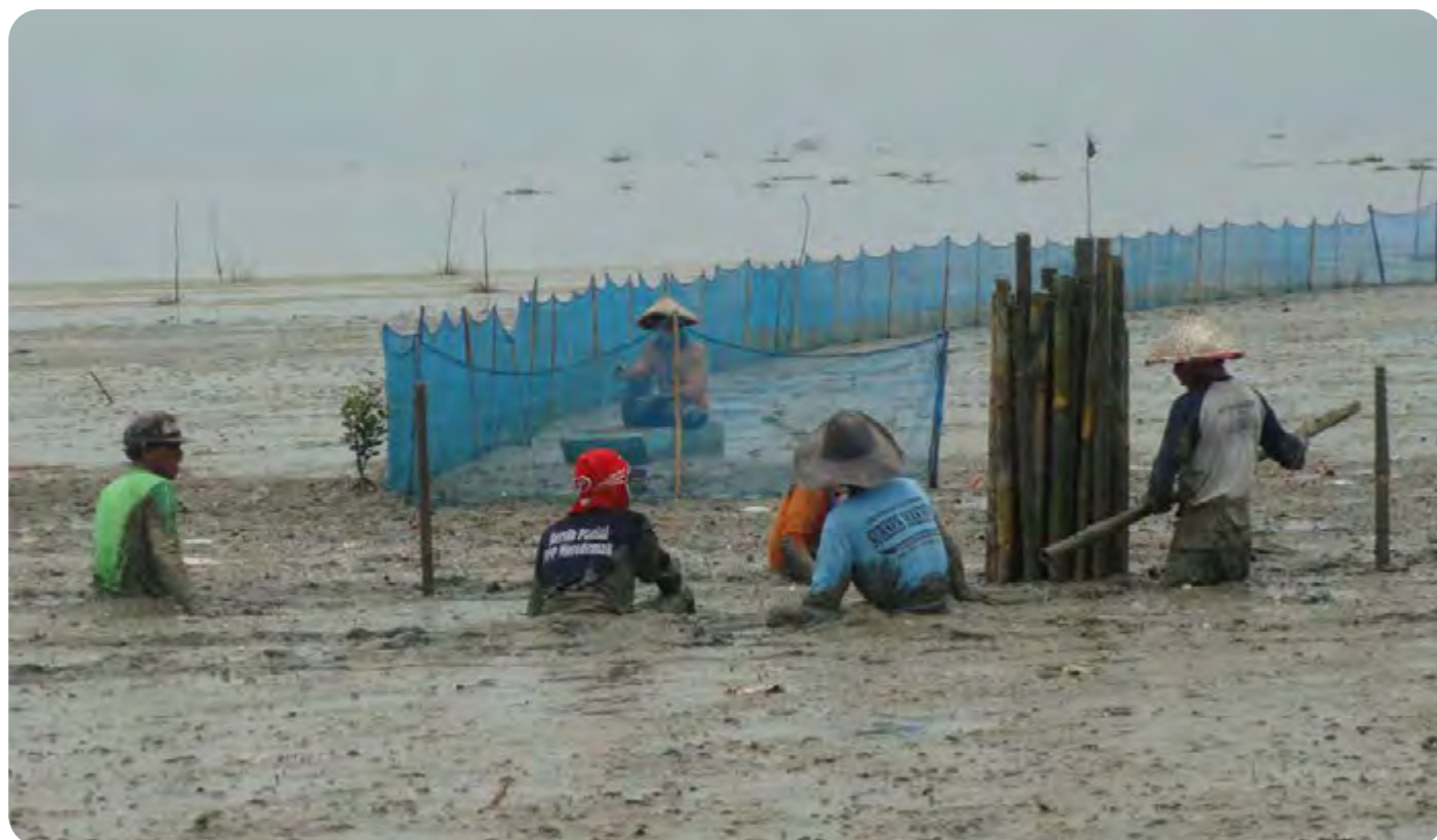
Community group installs a simple sediment trapping structure. © Kuswantoro
