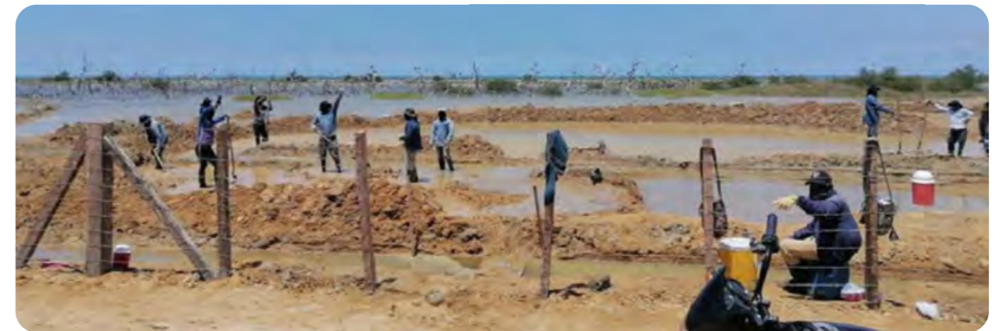
Local and ancestral knowledge informed the process of digging channels to secure water flows to and from the mangroves in Musichi. © Adriana Daza
